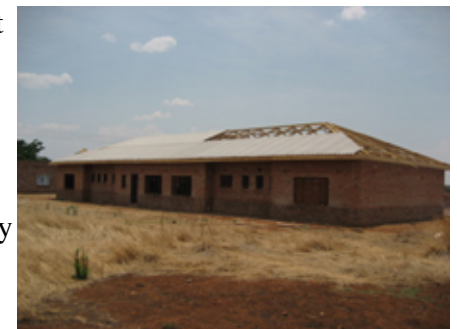
Zimbabwean house getting its first roof
